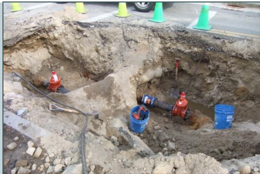
Valve Replacement on Reservoir Road
