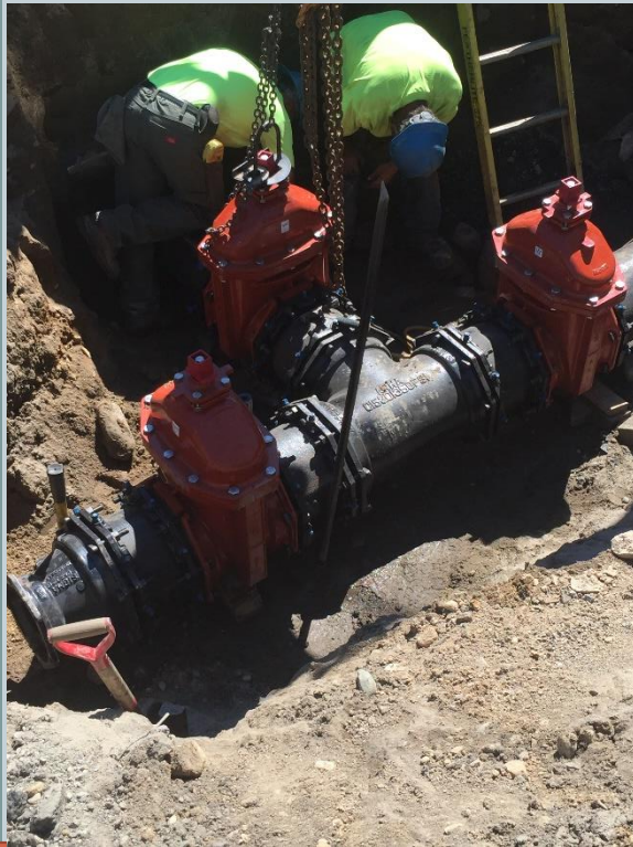
Installation of Tri-Valve at corner of North Main & Pascoag Main St.
