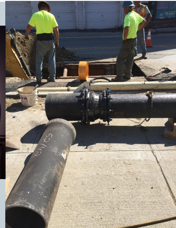
Installation of 14" to 12" Reducer Coupling on Pascoag Main St.
